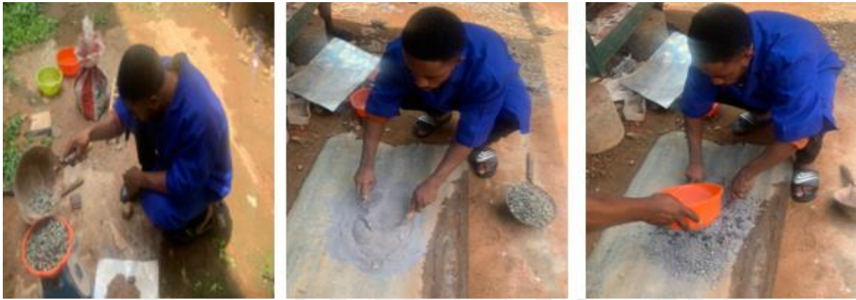
Figure 2: Mixing of the constituent materials
