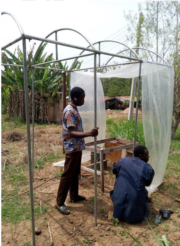
Figure 3: The greenhouse galvanized framework during construction
